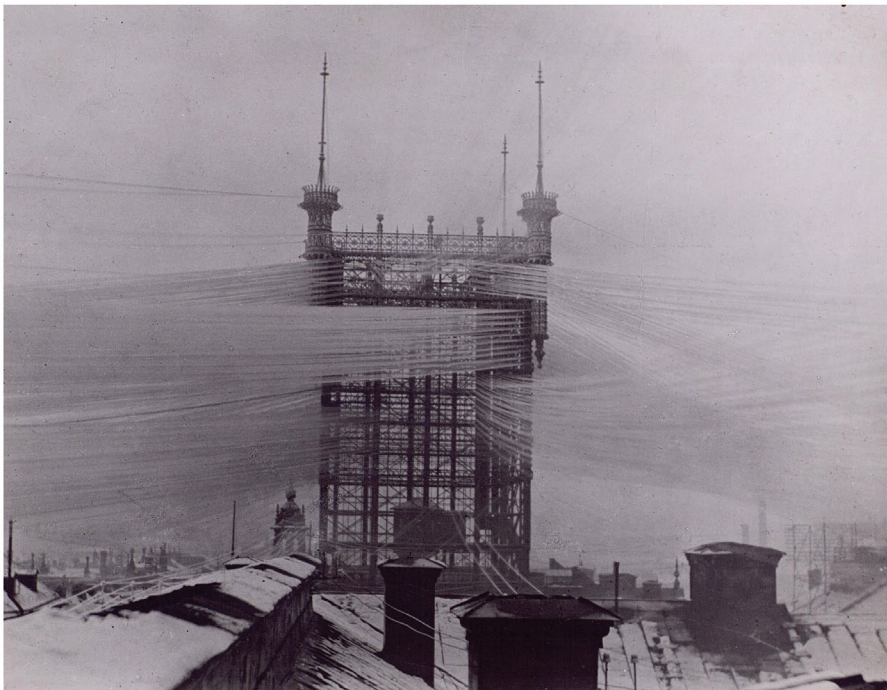
Figure 3. A telephone tower in Stockholm, Sweden with 5000 connected lines in use between 1887 and 1913. Source: Swedish National Museum of Science and Technology 2012.
