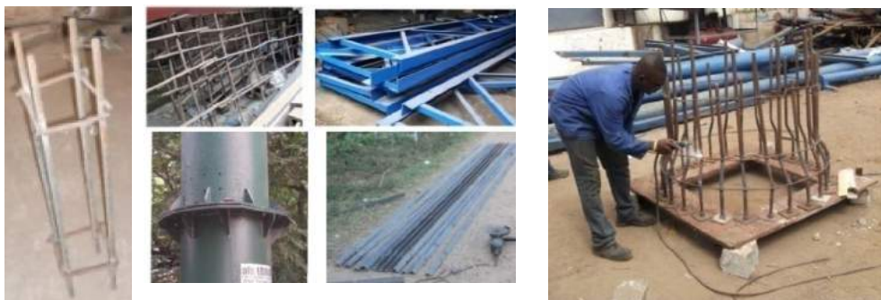
Hold down bolt Joint of two poles Angle Irons Construction of holding down bolt
